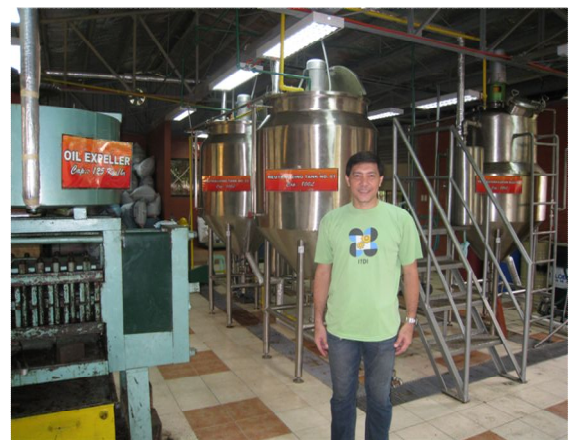
Jatropha Oil Biodiesel Processing Facility
