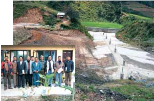
Name Mr. Rajesh Manandor Country Nepal Place of work Kathmandu Metropolitan City Training Course Solid Waste Management for Nepal ( Country training in 2004 ) Task Construction of semi aerobic landfill site in Sisdol
