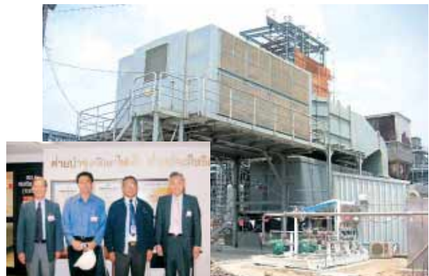
Name Mr. Chana Thitisak Country Thailand Place of work Electricity Generating Authority Training Course Automatic Control ( Group training in 2004 ) Task Construction of the electric power station for new airport
