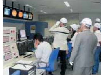
At the control room of Shin-Moji Incinerator Facility
