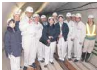
Visiting a site of installation of underground sewage pipes in Kitakyushu
