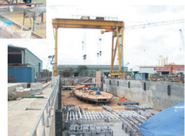
Dry Dock at Nam Trieu Shipping Industry Corp.
