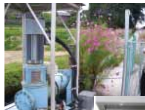
Plant for small-scale hydroelectric power generation in Taketa City, Oita Prefecture: 25 kW of electricity can be generated by using level differences of 8m.
