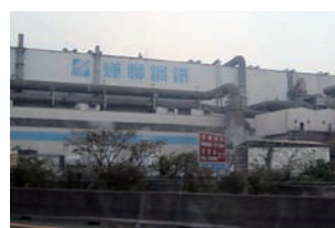
Electric Furnace Plant Yieh United Steel
