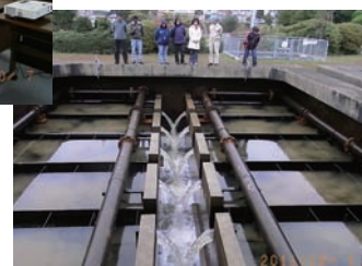
Observing the backwashing operation at Anoh Water Purification Plant, Kitakyushu
