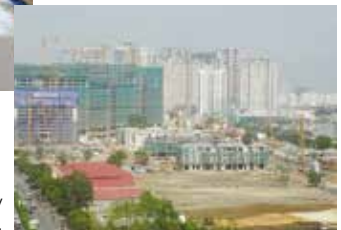
Ho Chi Minh City where construction rush is continuing.
