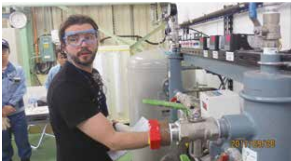
Actual practice on energy conservation by using an inverter
