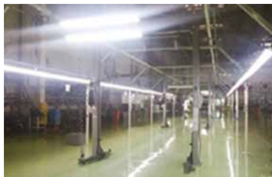
Example of improvement: 112V-fluorescent lamps were replaced with 72V-LED lamps.
