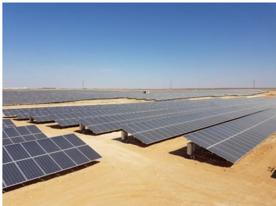
2) The following images shows (Saquer Ma'an) Power station
